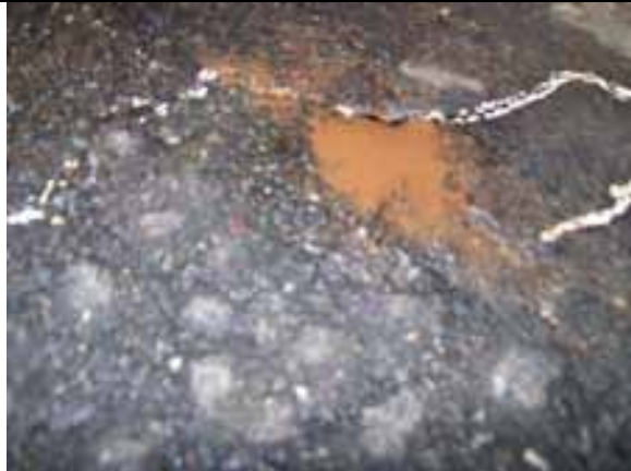
Asphalt cracks with fine base material pumping through
