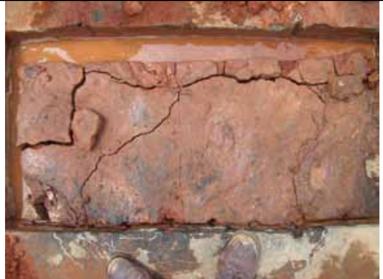
Side view of vertical HMA shear and plan view of CTB block before extraction
