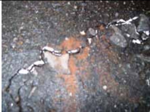
Asphalt cracks with fine base material pumping through
