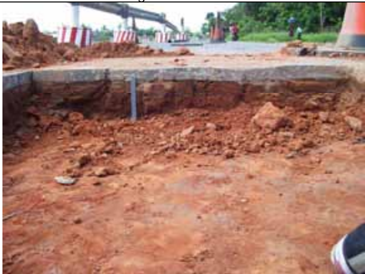
Pictorial views of diagnostic trench after excavation.
