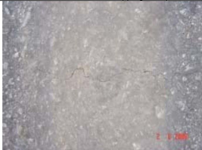
Transverse crack formation
