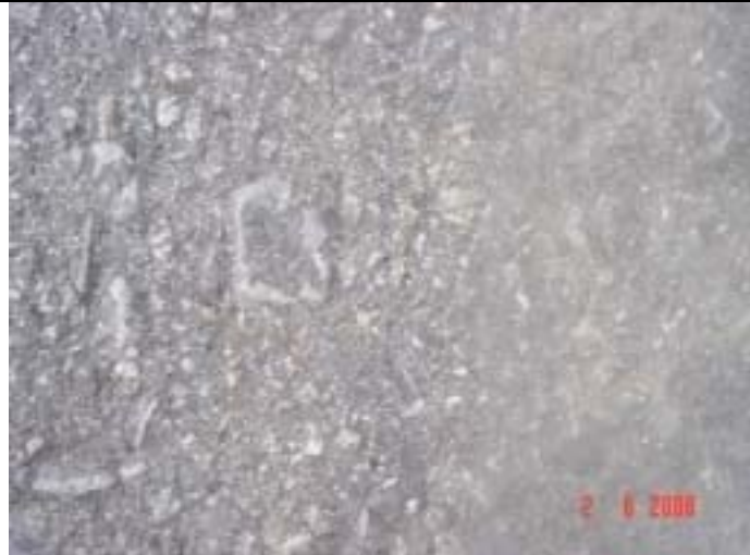
HMA surface texture. Note stripping of asphalt
