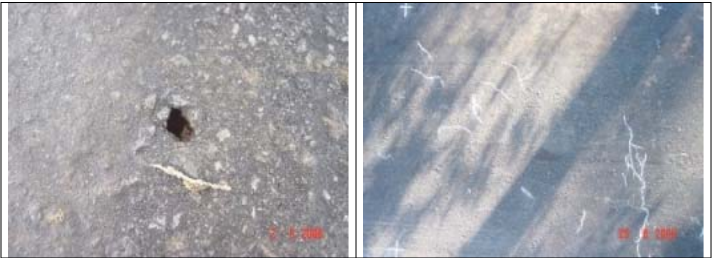
Asphalt surface texture. Plan view of test section
