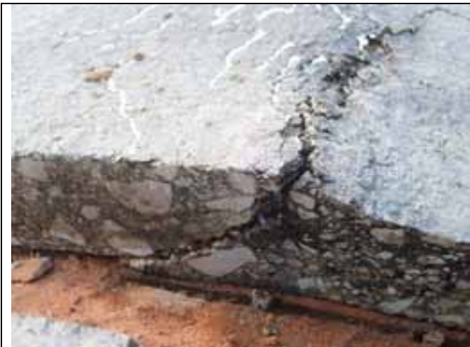
Close ups of HMA vertical shear
