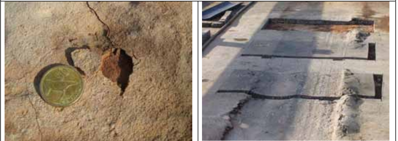
Close up of CTB surface after removal of HAM. Note smoothed surface texture.
