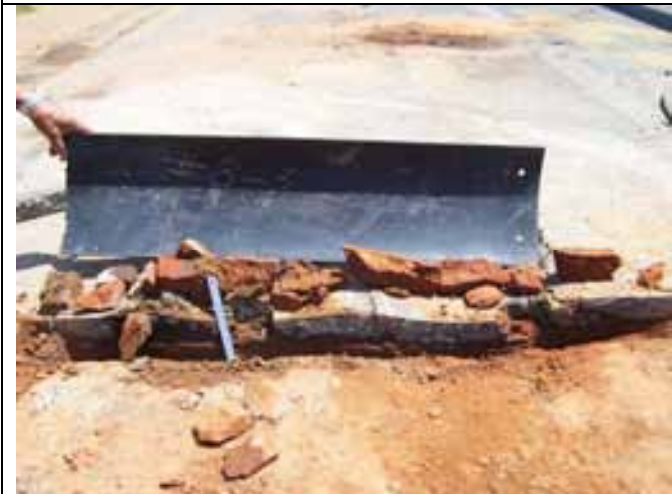
Removal of CTB fractures.
