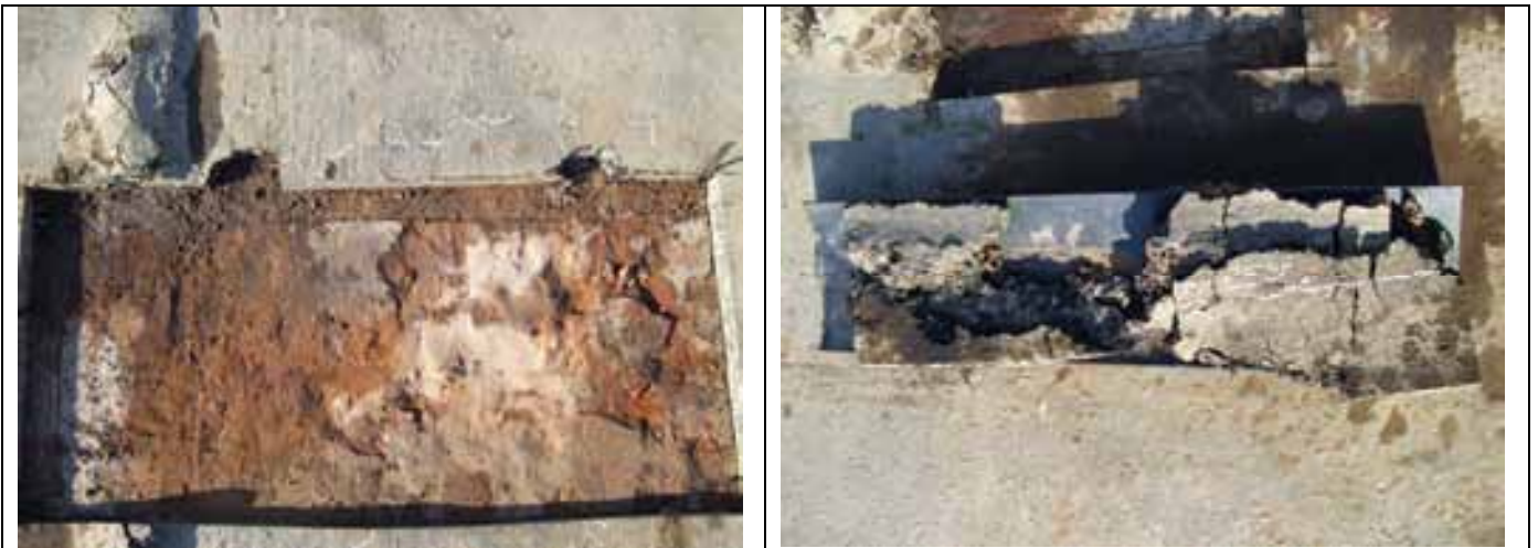
Plan view of CTB after removal of HMA mat
