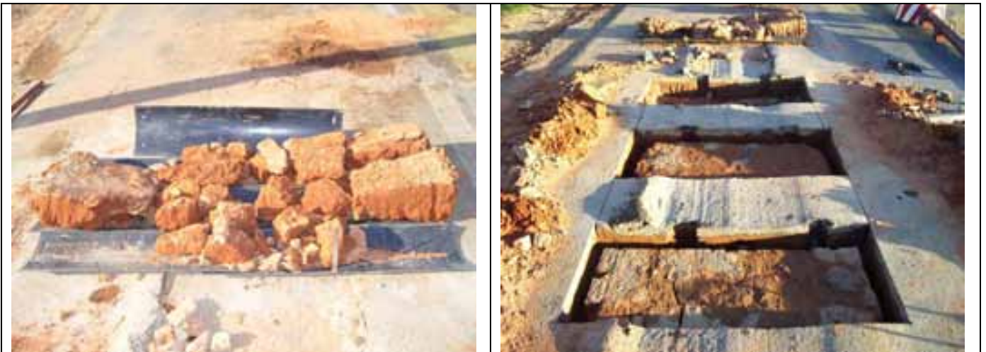
Removed CTB blocks and fractures. Overview of test pits.
