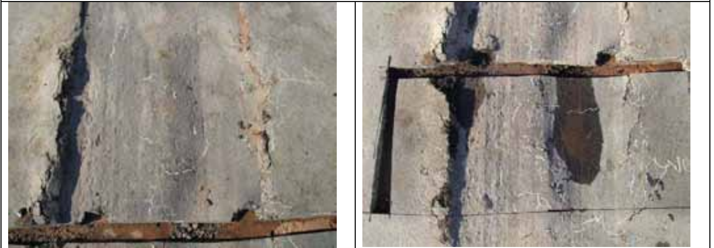
Plan views of test section before removal of HMA
