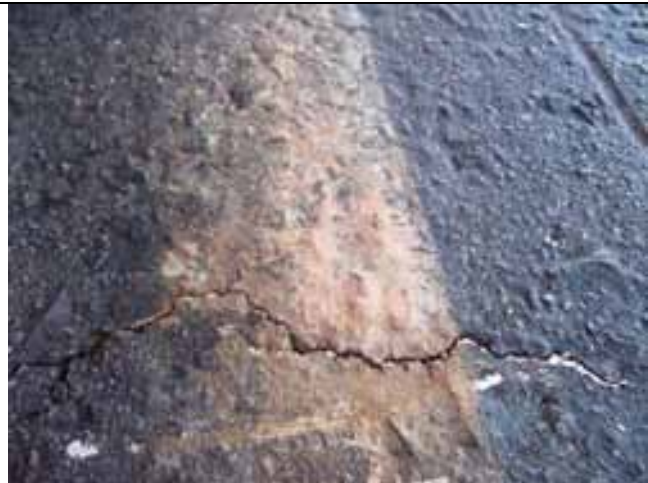
Close ups of material pumping through cracks in asphalt
